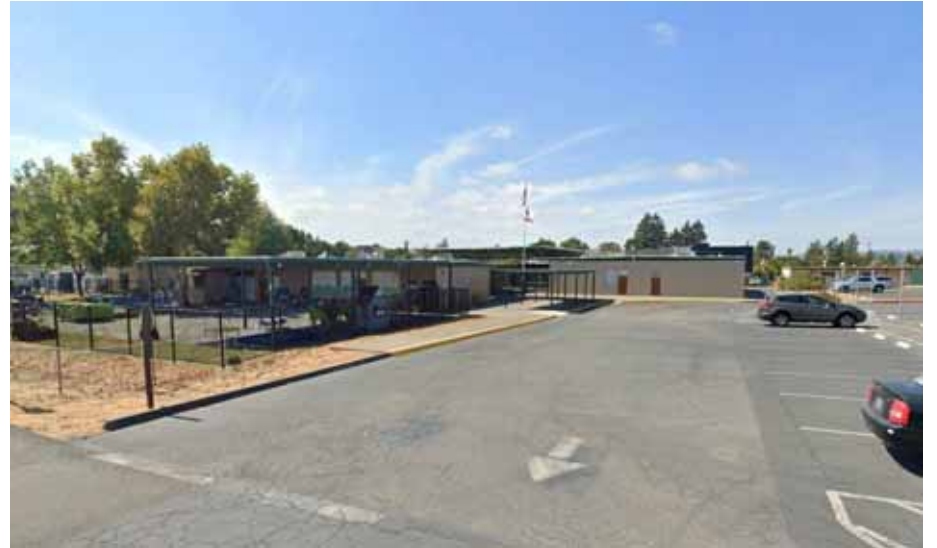
View west from Subject Property
